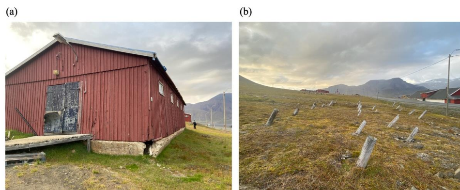
Figure 1. The impact of the thawing permafrost on construction in Svalbard. (a) Warehouse damaged, and (b) slanted house foundation due to permafrost thawing.
